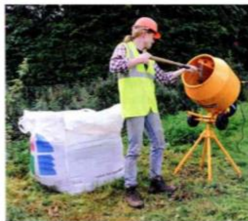
Mixing sand, cement and water to make mortar.
